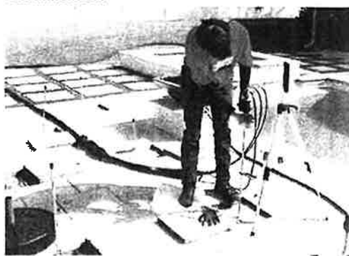
Paver Pool Deck Soil Stabilization
